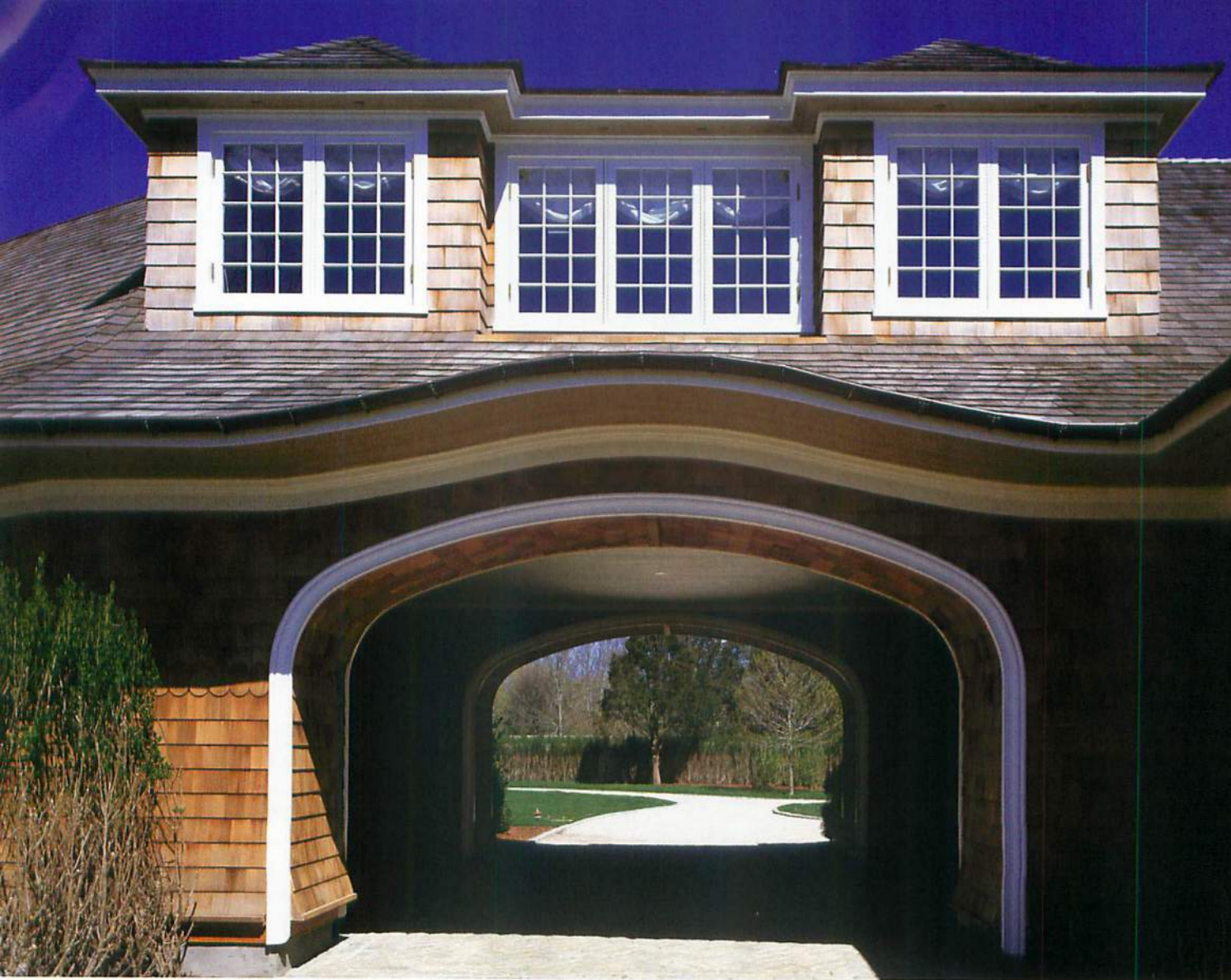
Above: Porte cocheres are once again in favor, this one leads to the five car garage housing specimen cars, note the eyebrow soffit mimicking the opening below.
